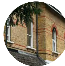
Changes in brickwork
