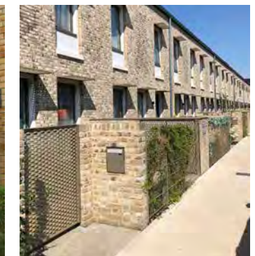
Integrated bin and cycle storage
