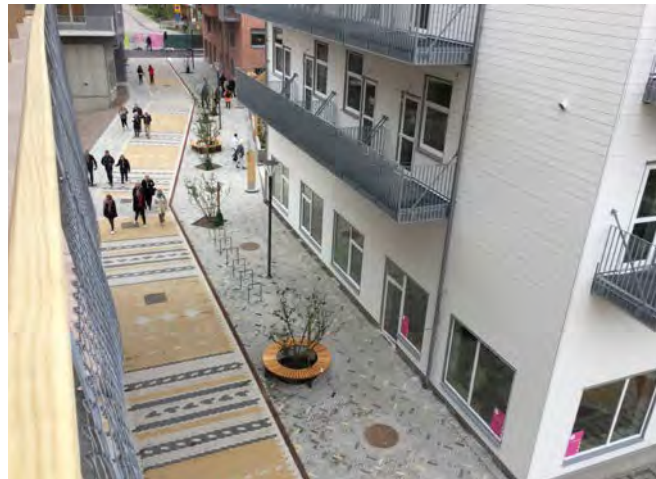
Use of patterns, materials and detailing in the public realm to create attractive pedestrian-priority streets that lead people through the neighbourhood.
