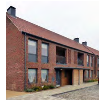
Inset balconies on maisonette upper floors
