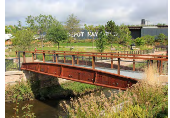
Using the design and materiality of bridges as important connection points and features.
