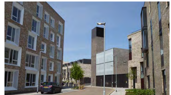
Energy Centre co-located with supermarket fridges and designed as marker building in street
