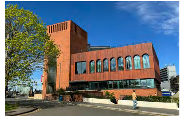
Landmark building in prominent location
