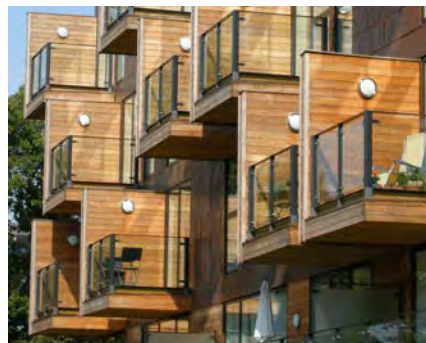
Privacy screens on protruding balconies
