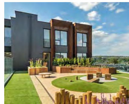
Shared roof terrace space sheltered from prevailing winds
