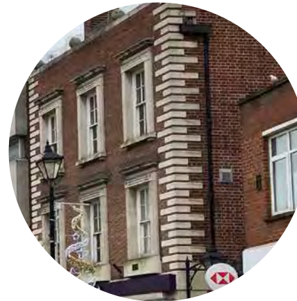
Corner brickwork detailing and brick variation
